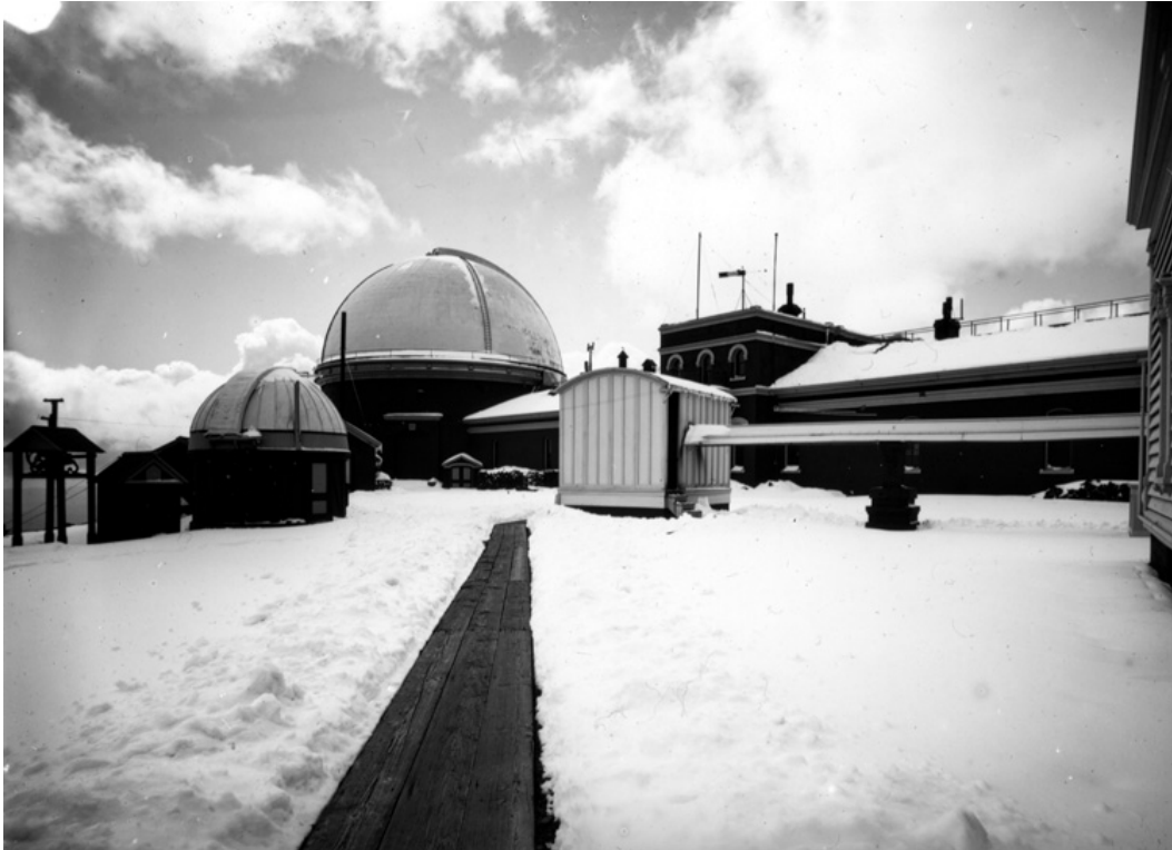
Figure 3: The photographic house of the photoheliograph is at center, with its horizontal tube extending north toward the heliostat. Dome of the 36-inch refractor is in the background. View is looking southwest (no date, but between 1888 and 1907). Photo courtesy of Darrell Severinsen, Lick Observatory.
