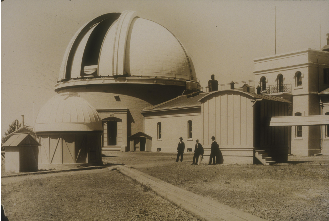
Figure 5: The photographic house of the photoheliograph is at right, with its horizontal tube extending north toward the heliostat. Dome of the 36-inch refractor is in the background. View is looking southwest (no date, but between 1888 and 1907). Photo courtesy of Darrell Severinsen, Lick Observatory.
